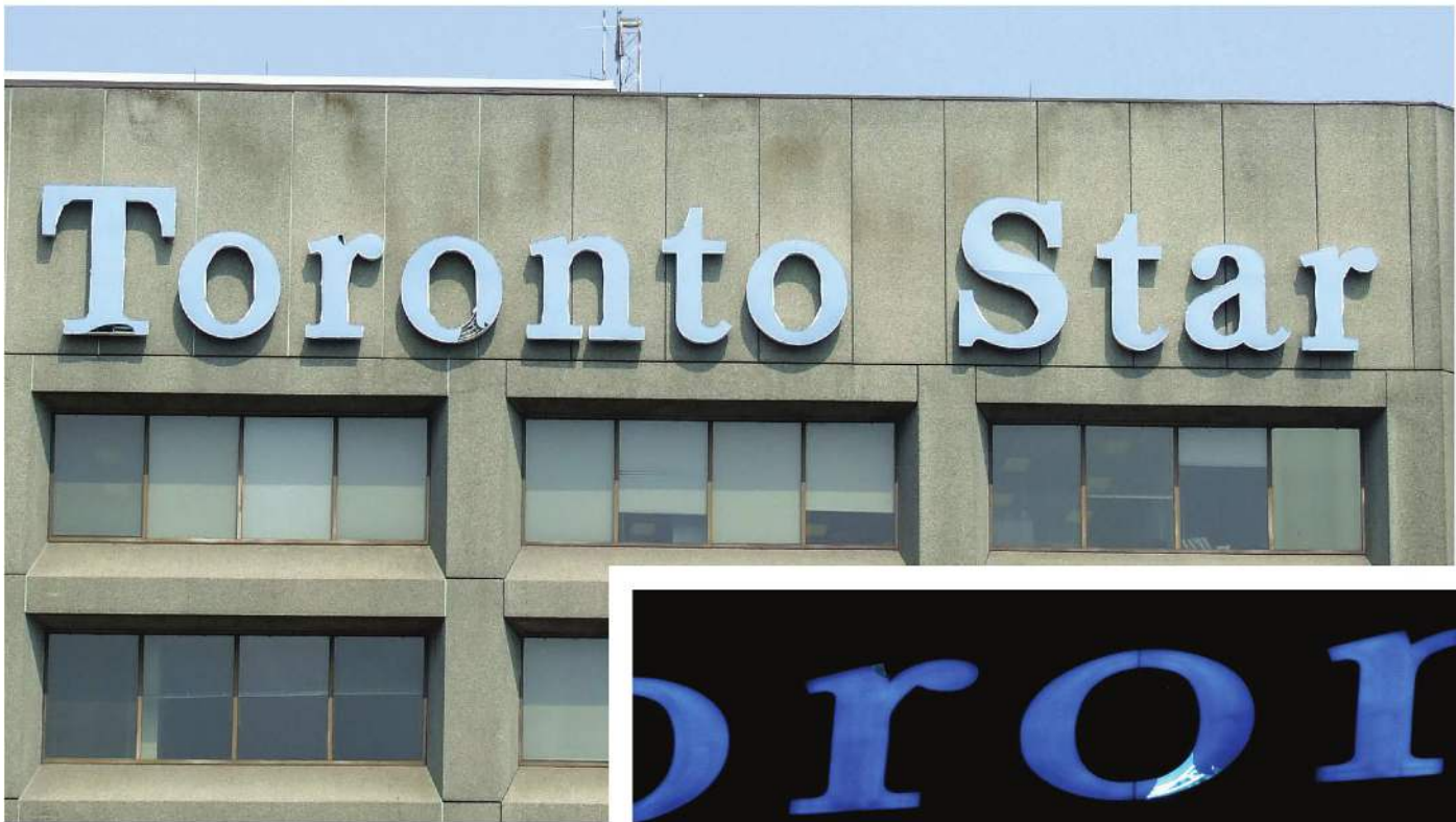
Prior to their LED retrofit in 2014, the sign's steel letters were battered and rusty and had large holes in them.
